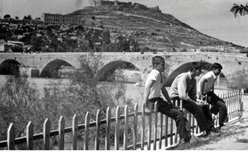
Taş Köprü / Silifke / Mersin 1967
